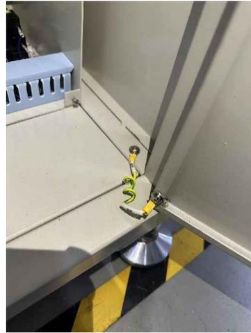
Picture 16 Hazard 2.3, Image 2, PE cables
