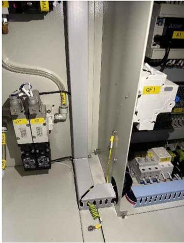
Picture 15 Hazard 2.3, Image 1, PE cables
